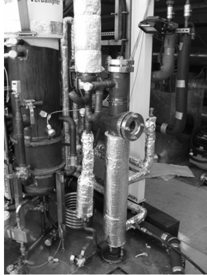
Fig. 7: Generator B III after the reconstruction of the DACM (photo: zafh.net).
