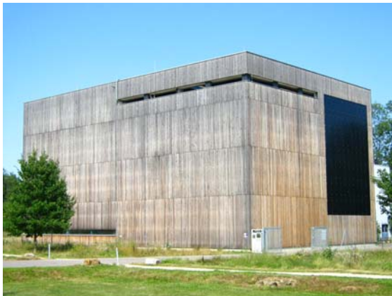
Fig.5: BIPV in Scharnhäuser Park Ostfildern with 70 dark backsheet modules STM200F (SunTechnics).
