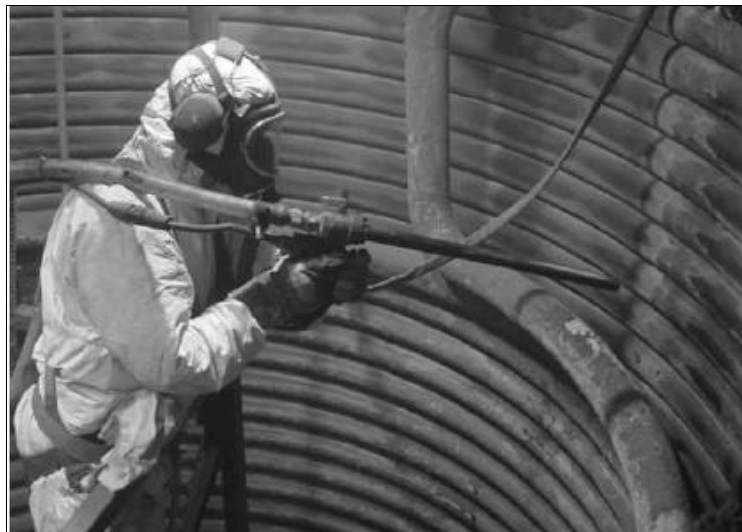
Fig.4. Manual boiler cleaning
