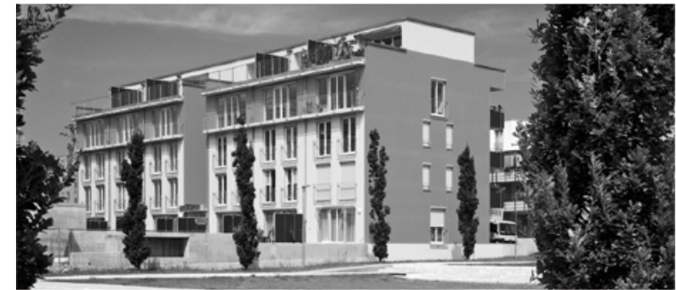
Figure 5: Photograph of multi-family building with detailed monitoring results.
