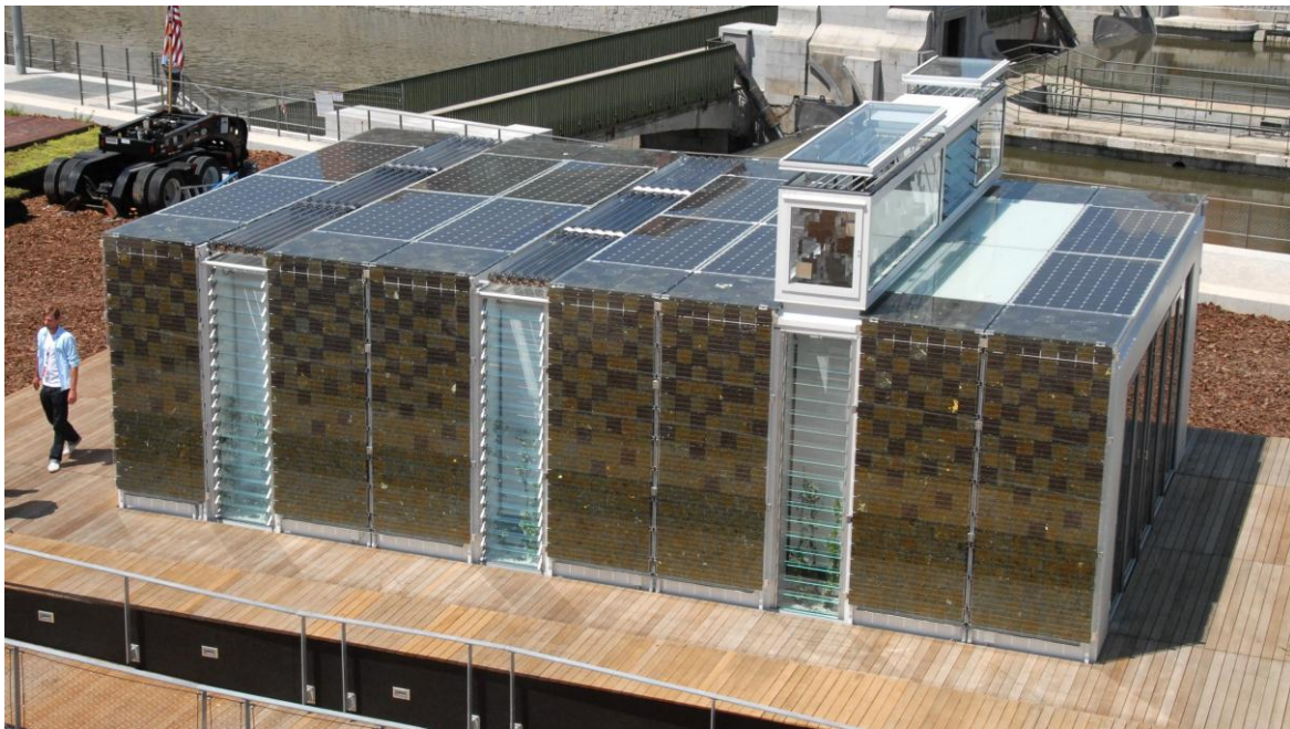
Figure 2: Solar Decathlon Building with PVT roof.
